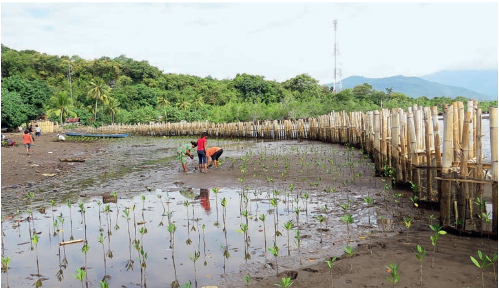
Figure 3-6 Mangrove rehabilitation using bamboo for sediment trapping by local community in Banten, Indonesia. (Photo by Virni Arifanti)
