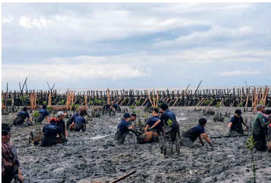
Figure 4-8 Mangrove replanting program using eco-engineered structure as a wave breaker to reduce erosion impact in Sungai Haji Dorani, Selangor. (Photo by Tariq Mubarak Husin)
